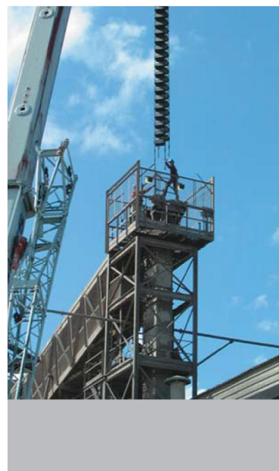
Figure 17: quick and simple assembly of a HEKO endless chain strand
